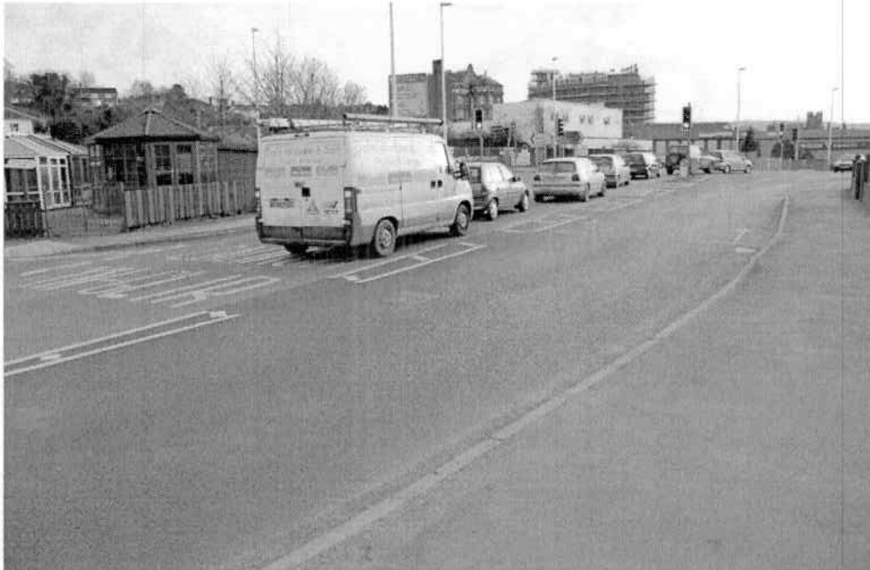
Photograph 3.2: Showing the right turn lane and the 'keep clear' markings over Sheaf Street.
